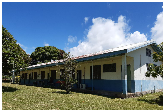
Training facility at Northern Provincial Hospital, Santo
