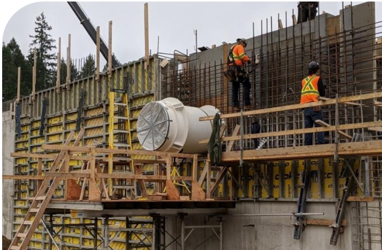
Comox Valley Regional District Water Treatment Project.
