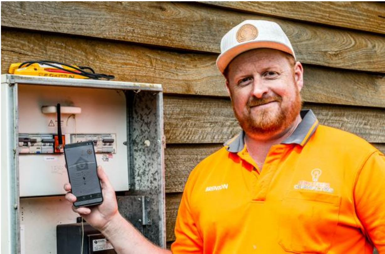
Figure 16 Local electrician installing a Wattwatchers device on a switchboard in Heyfield.
