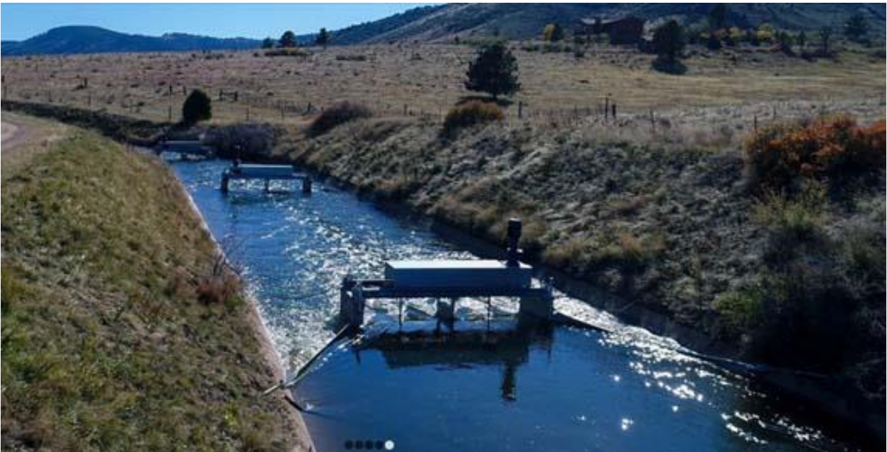
Figure 11 Hydro turbines at work along an irrigation channel (each produces 10-25kW)
