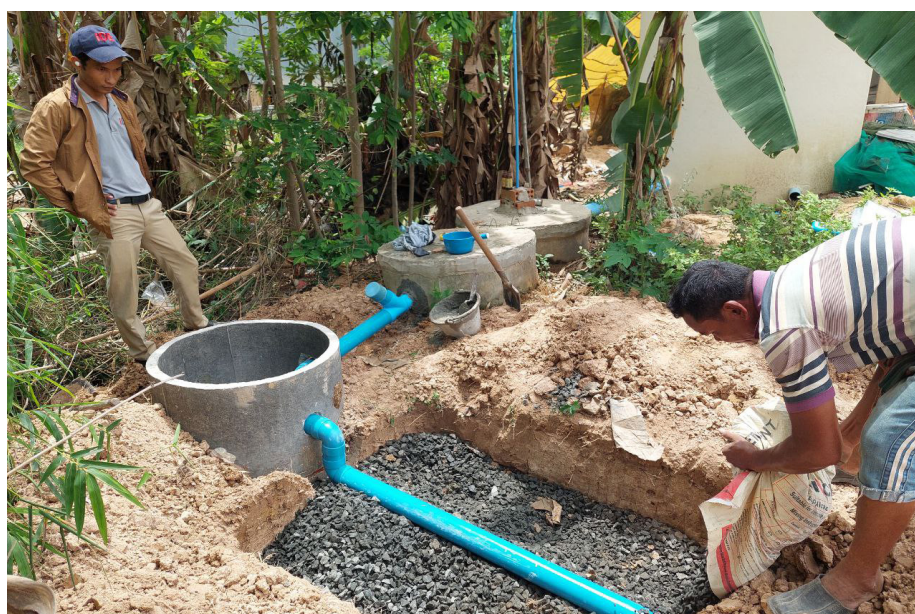
A sanitation business labourer installs an iDE-designed latrine upgrade to maintain toilet functionality in high groundwater and dense, saturated soil. He adds gravel to the leach field to provide preliminary treatment of the wastewater and increase surface area for improved infiltration
