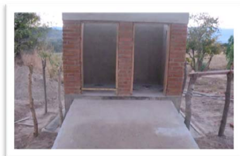
Figure 4: Ramps in school toilets in Malawi enable access for pupils with a disability. Photo: WaterAid
